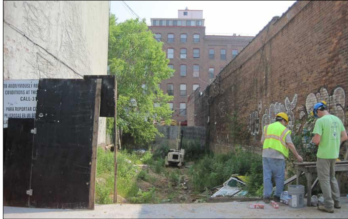
A brownfield site in Brooklyn. Photo courtesy of Hydro Tech Environmental, Corp.
