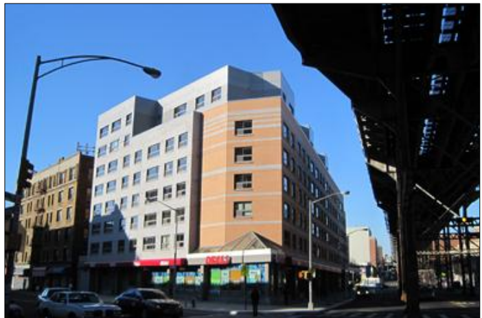
Redevelopment of the brownfield site in Brooklyn led to a LEED silver-certified building with affordable housing and retail space. Photo courtesy of the Mayor's Office of Environmental Remediation.
